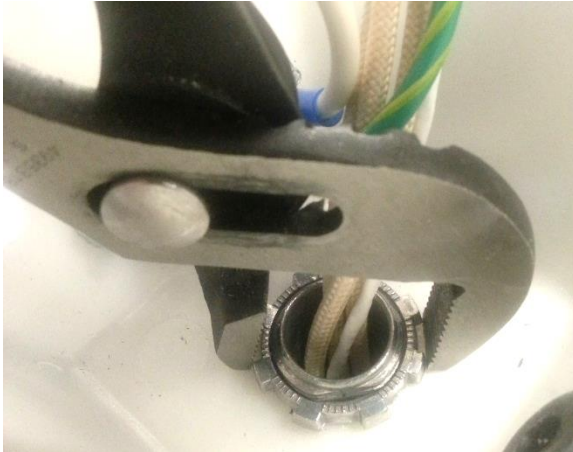
Screw on Conduit Retaining Nut using Pliers
